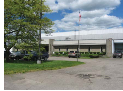
Crescent Manufacturing’s Eagle Drive headquarters
