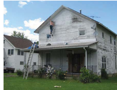
Addressing deferred maintenance at a Spruce Street home
